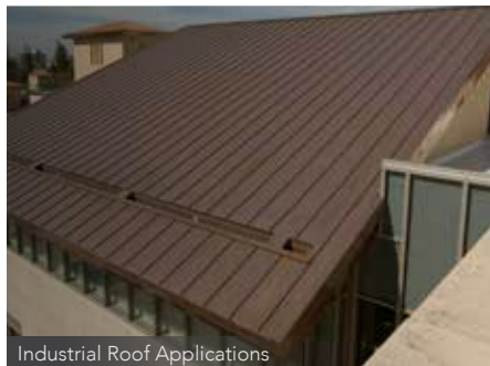
Industrial Roof Applications
